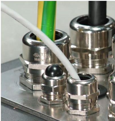
Figure 47: Tighten cable glands
