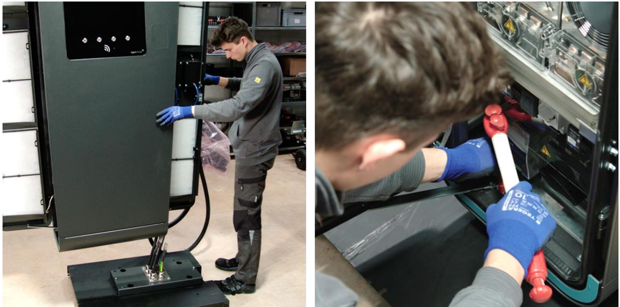
Figure 48: Positioning and attaching the HYC400 on the base
